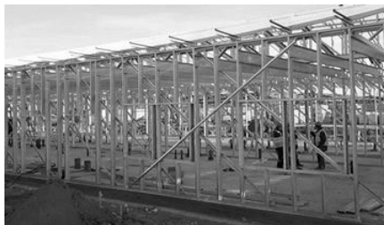
Fig.3. Light steel thin-walled structures
