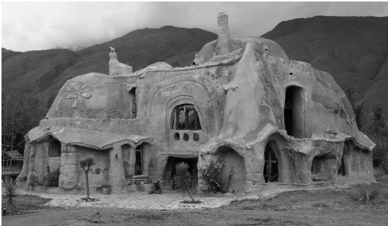
Fig. 3. Casa Terracotta, Spain
