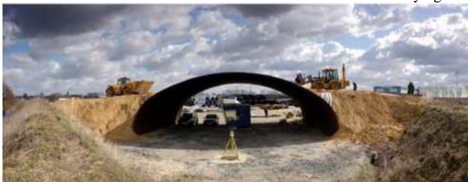
Fig. 1. Example of soil-steel flexible SuperCor structure [3]
