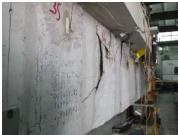
Fig. 5. Beam failure – telescopic effect and debonding of the middle PBO strip
