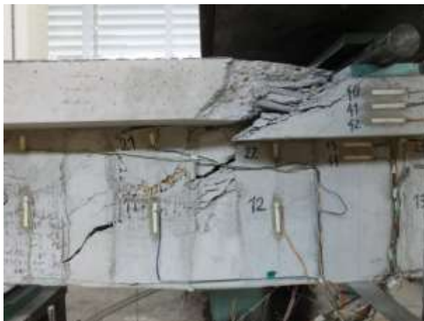
Fig. 4. Beam failure – destructive diagonal crack, rotation of the anchorage and PBO mesh debonding
