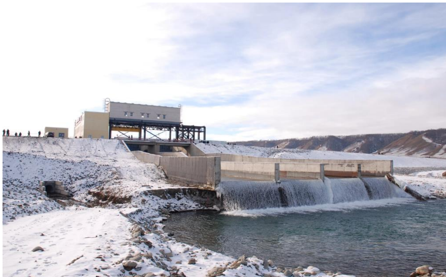
Fig.3 Small hydroelectric power station on the Bolshoy Zelenchuk river (the Karachay-Cherkess Republic)
