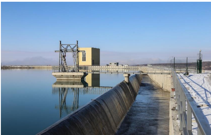
Fig. 6. Zaragizhskaya small hydroelectric power station in the Kabardino-Balkaria Republic
