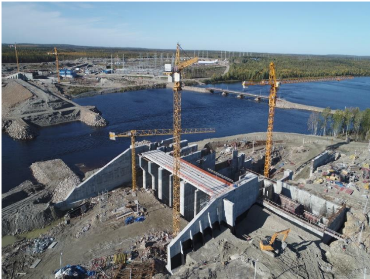
Fig.5. Construction of Beloporzhskaya small hydroelectric power station in Karelia
